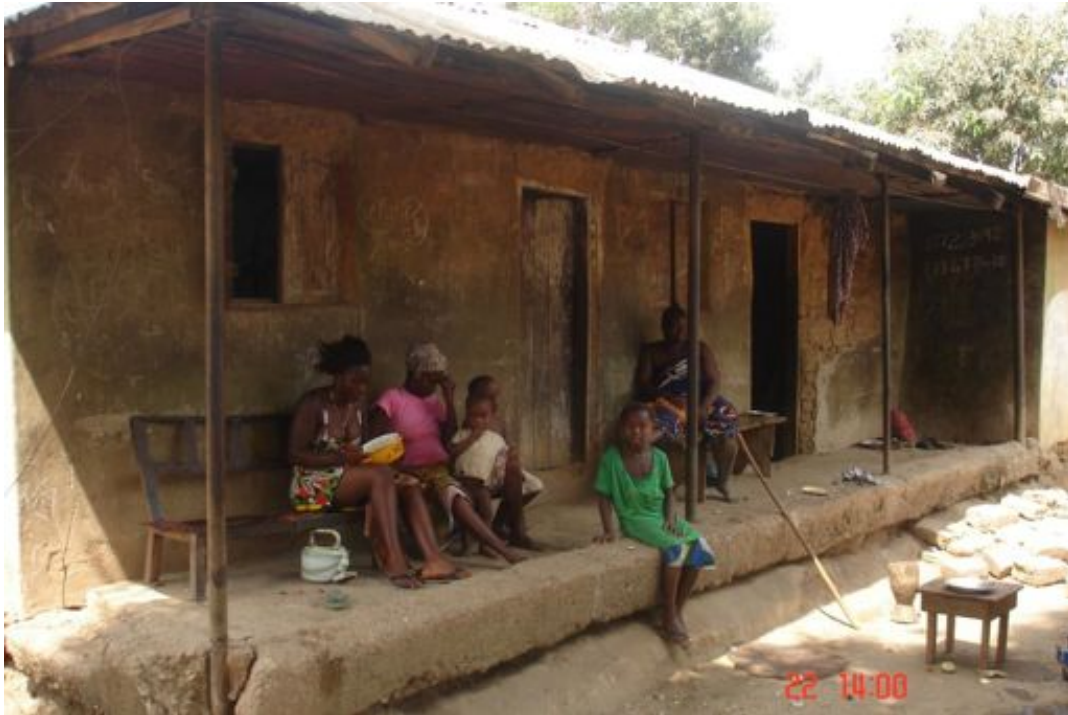
Old Structure B-18 Sulaiman Kamara c/o Adama Kamara 7 Bedrooms
