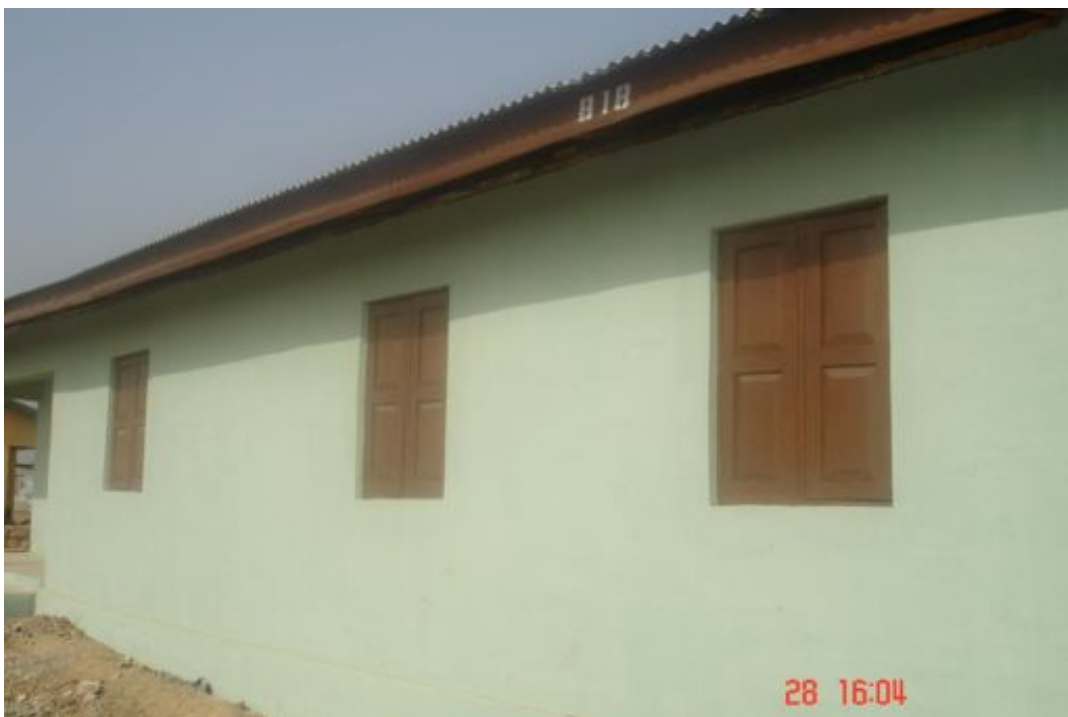
New Structure B-18 Sulaiman Kamara c/o Adama Kamara 7 Bedrooms
