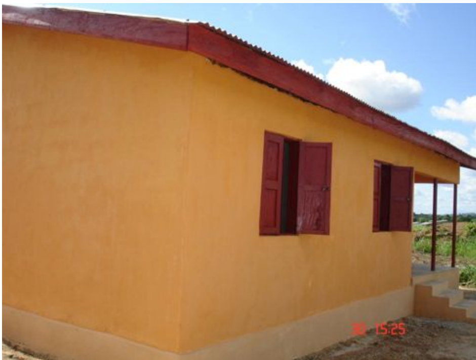
New Structure: C 61 -5 Komba Paima c/o Sia Komba 4 Bedroom
