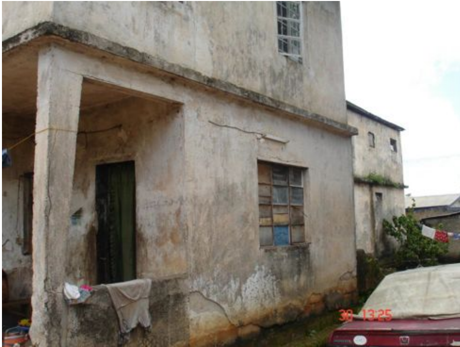
Old Structure: C 61 6 Komba Paima c/o Sia Komba 4 Bedroom
