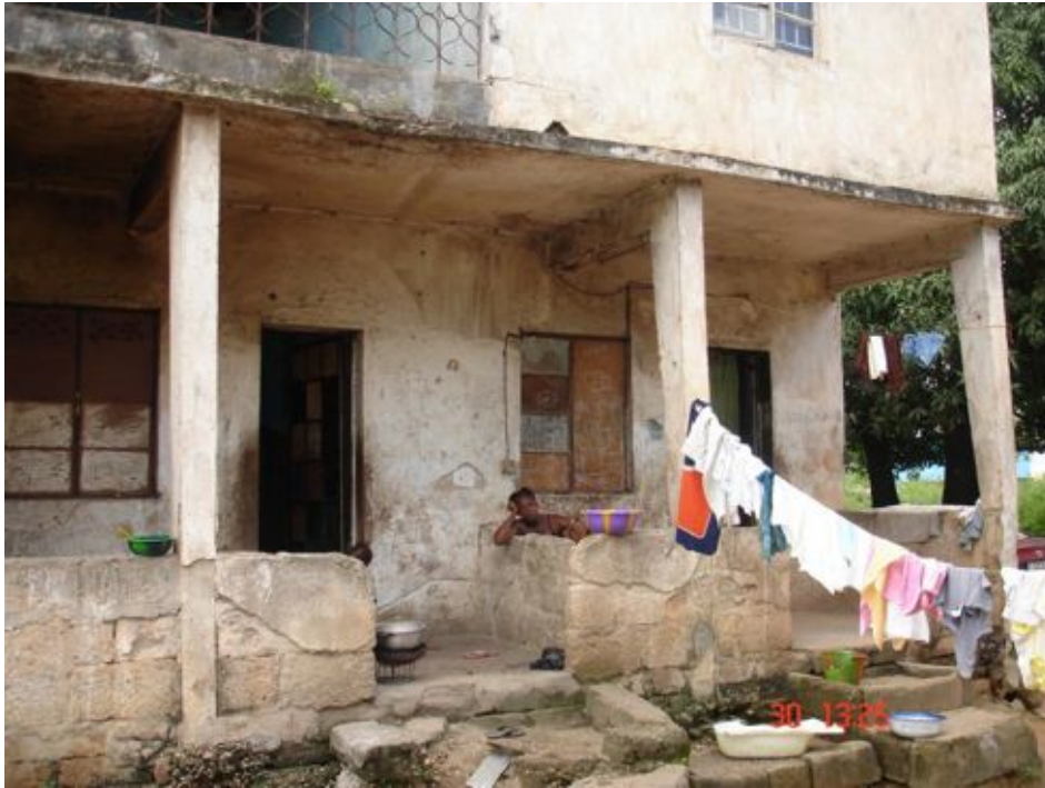
Old Structure: C 61 -5 Komba Paima c/o Sia Komba 4 Bedroom
