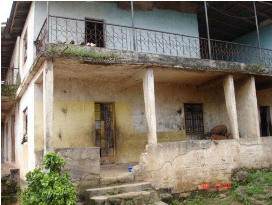
Old Structure: C 61 -4 Komba Paima c/o Sia Komba 4 Bedroom
