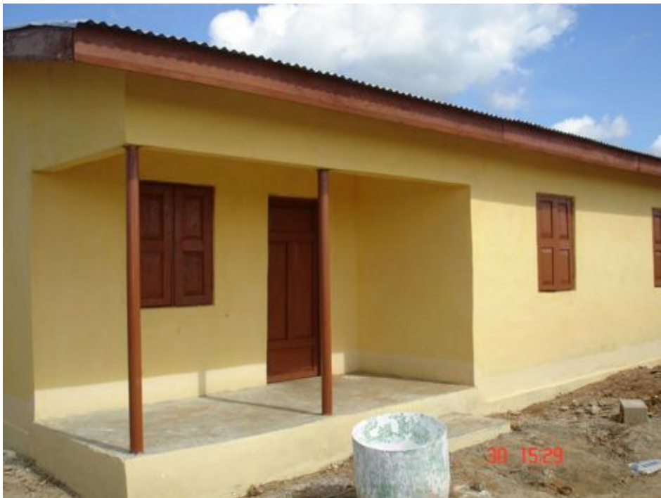
New Structure: C 61 6 Komba Paima c/o Sia Komba 4 Bedroom
