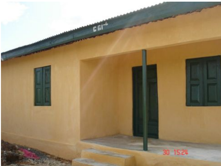
New Structure: C 61 -4 Komba Paima c/o Sia Komba 4 Bedroom
